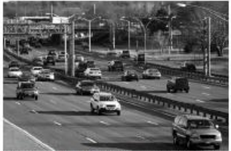
(b) Divided multilane highway in a suburban environment.
