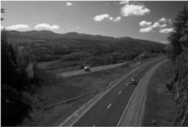
(a) Divided multilane highway in a rural environment.
