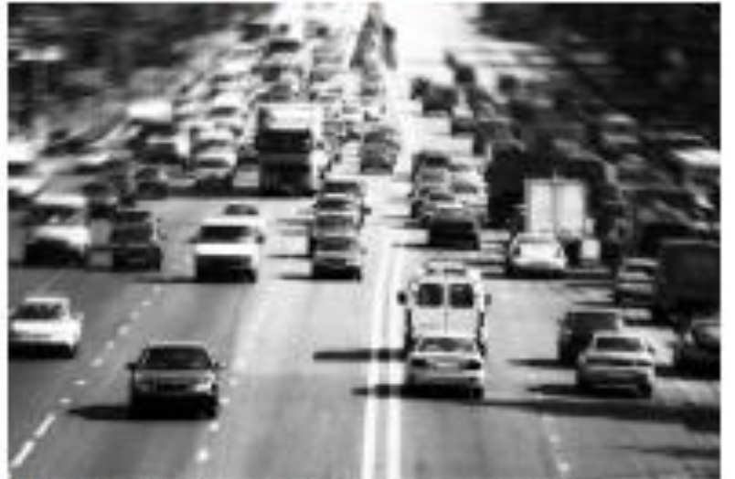
(d) Undivided multilane highway in a suburban environment.
